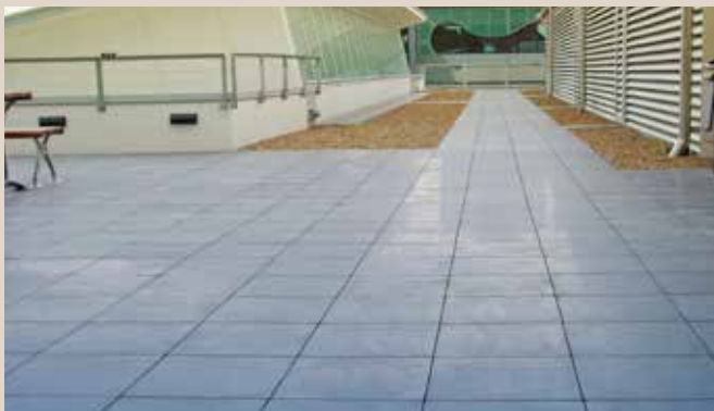
Chatswood Police Station, Australia
